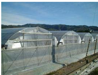
Fig.1 Photograph of greenhouse
