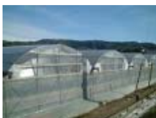
Fig.1 photograph of greenhouse
